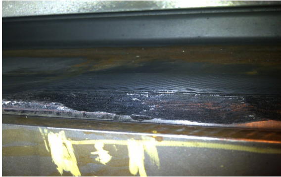
Figure 19. Slot 24 ready for weld repair
